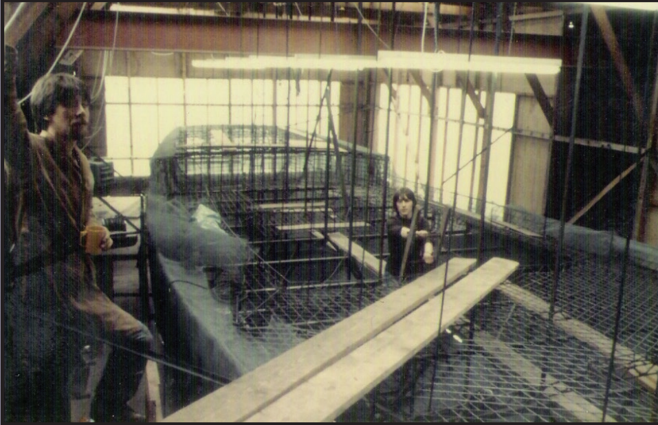
Building armature: making the iron frame of the ferro cement boat and then weaving 10 layers of chicken wire onto it.
